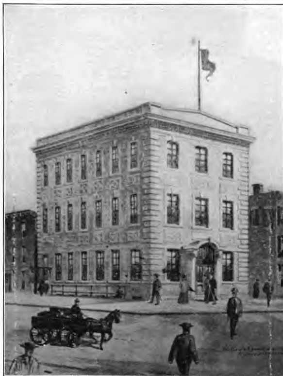
THE BUILDING—The Basement contains six rooms, all for Medical Work. The First Floor is the Auditorium the Second for our different schools and the Third for our Offices and Reading Room.
