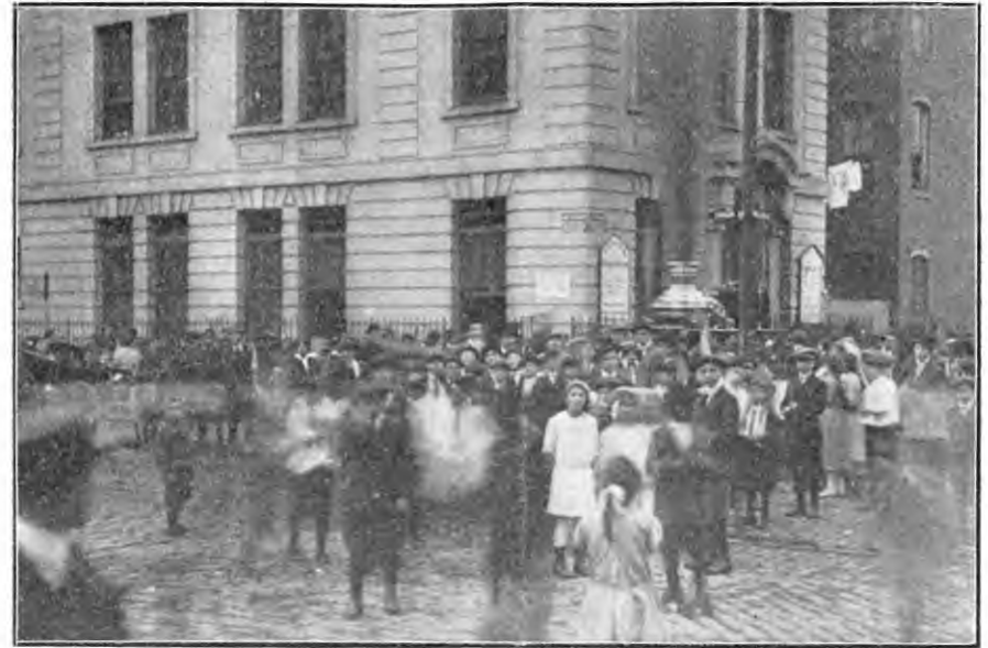
Pumping Out the Water From the Basement of Our Building
