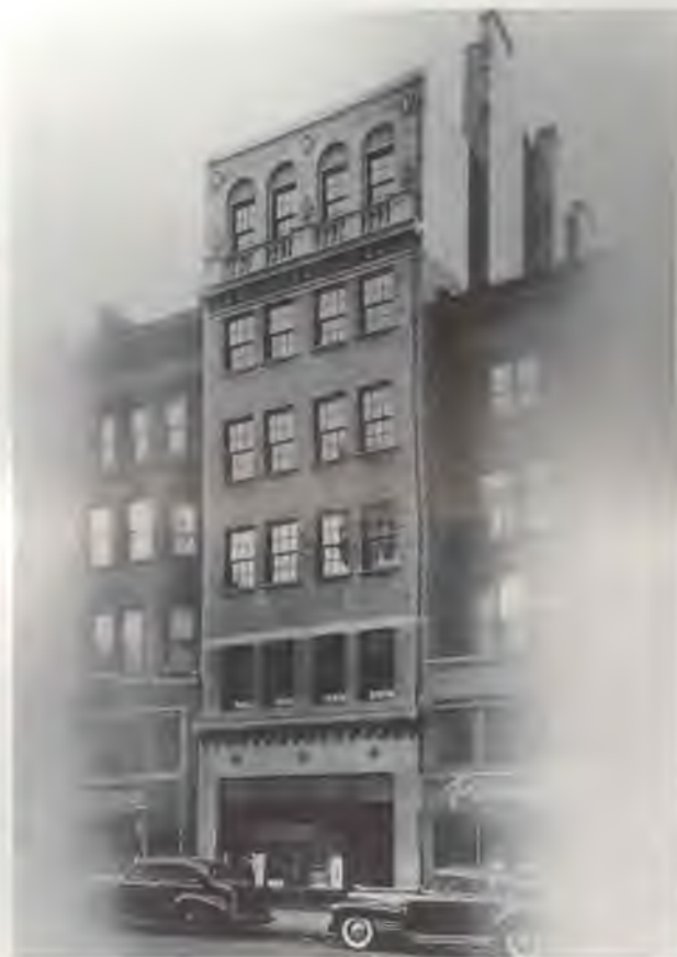
This building in New York City once served as CPM’s headquarters. The headquarters moved to Charlotte, North Carolina in 1988.
